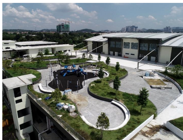
Photo Caption: MMC PLSB is the main contractor for the construction of Langat Centralised Sewage Treatment Plant that has the capacity of 920,000 population equivalent covering a total of 77.6 sq km catchment area starting from Cheras Batu 11 to Kajang. It is designed to
